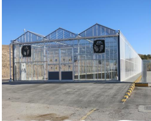
Install the first of its kind solar sludge drying greenhouse in Mutah WWTP
