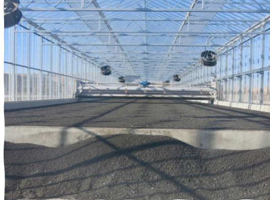
Install the first of its kind solar sludge drying greenhouse in Mutah WWTP
