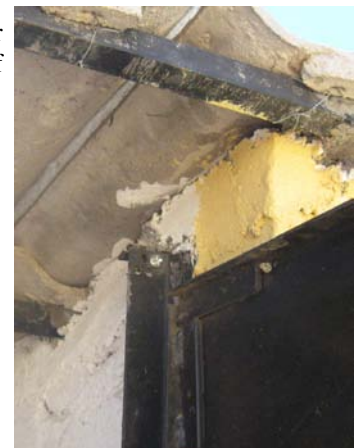
south door roof
