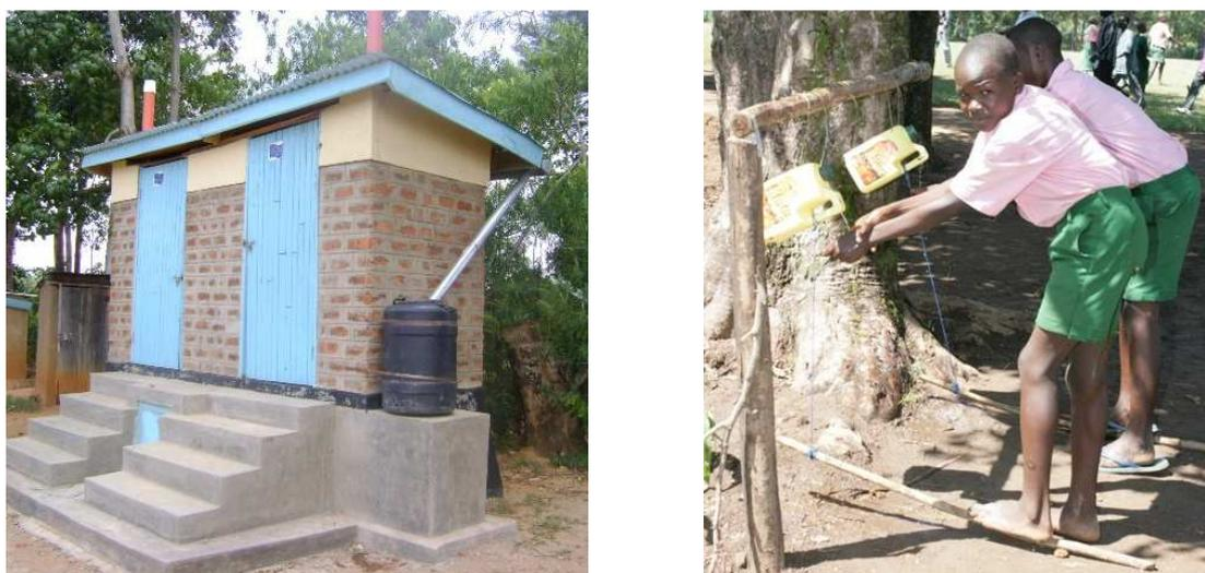
**Fig 1.** Left: UDDT school toilet with hand-wash unit connected to rainwater harvesting; right: Pupils in Khaimba Primary School wash their hands with newly installed tippy taps (source: C. Rieck).
