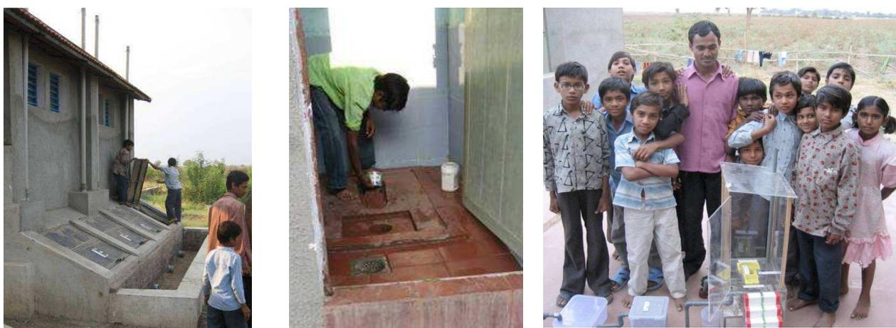
**Fig 2.** UDDTs at the sanitation facility of the primary school at Rayka village. Left: Faeces dehydration chambers with vent pipes; middle: faeces are sprinkled with dry material, e.g. ash/rice husk; right: ‘Young scientists’ who received first prize for the ecosan school toilet model (source: ESF).
