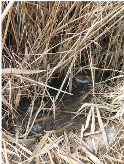
**Fig. 9:** Overloaded, water-logged reed bed towards outlet section of reed bed (source: E. v. Münch, Jan. 2009)
