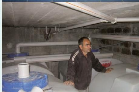
The caretaker in the basement where four urine tanks (each 2 m<sup>3</sup>) are installed (photo by AWHHE)
