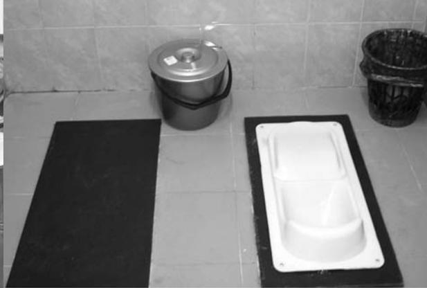
*Restroom with the squatting slab on the right. When the right faeces chamber is full, the slab has to be switched to the left side and the right place will be closed*
