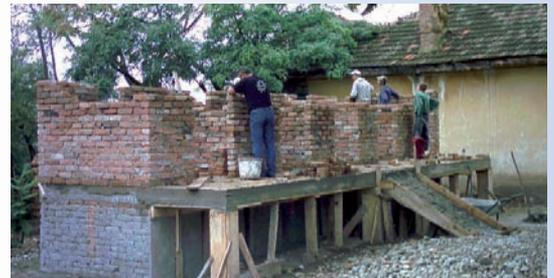
Construction of the toilet building with local material
