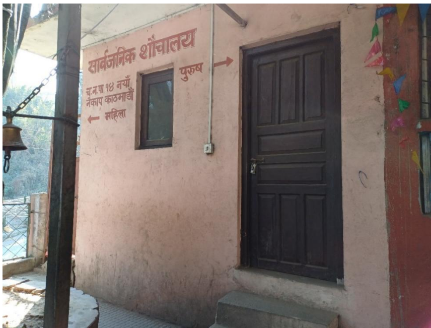
Figure 13: Public toilet and its status at Naya Naikap .
