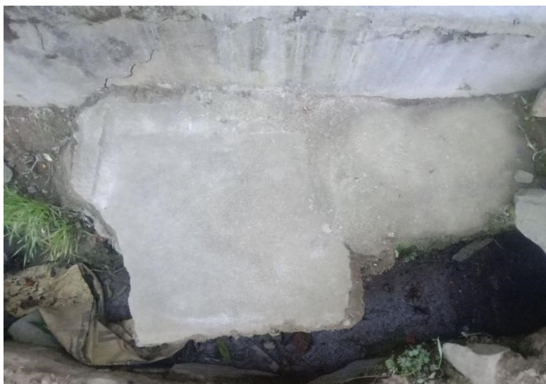
Figure 5: Sludge disposal in an open drain in Chandragiri Municipality.
