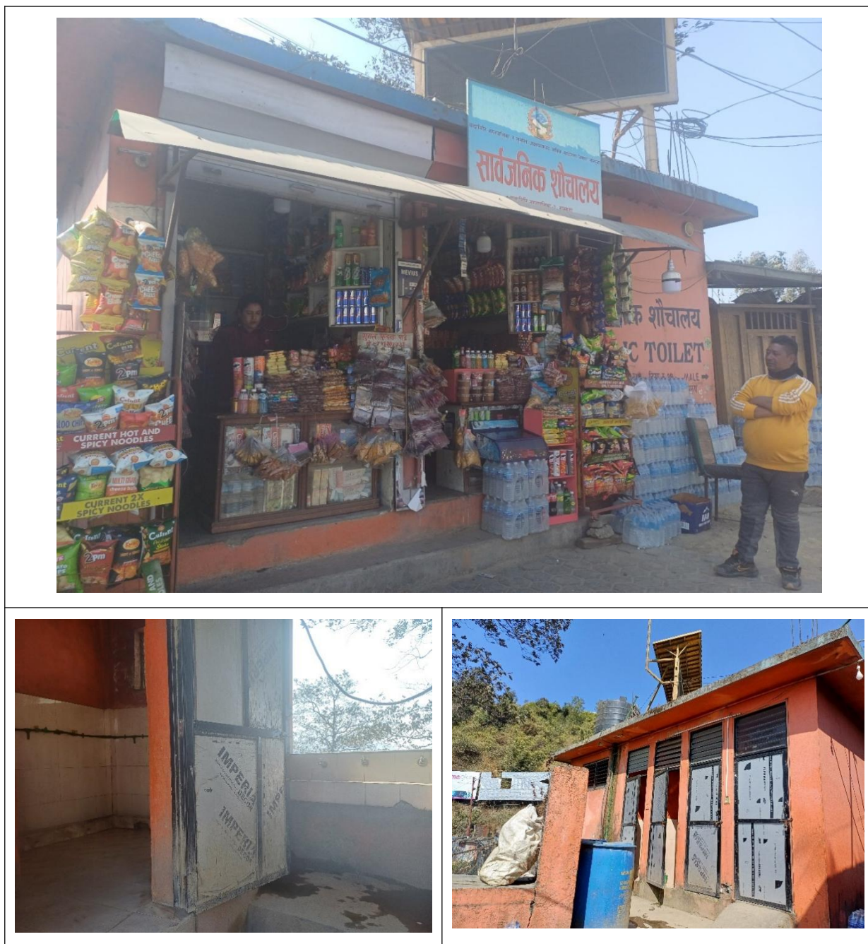
Figure 12: Public toilet at its status located at Nagdhunga Buspark.
