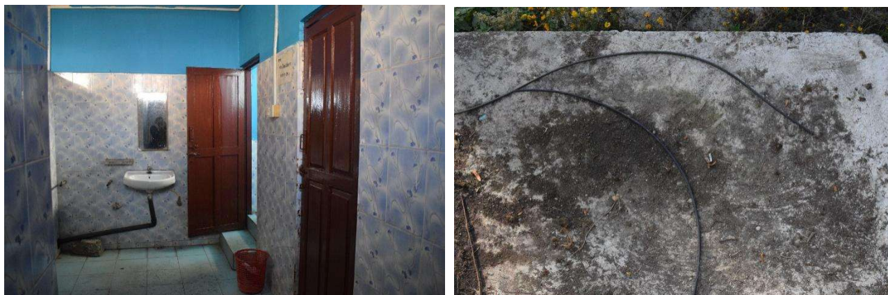
Figure 6: Public toilet near buspark area.
