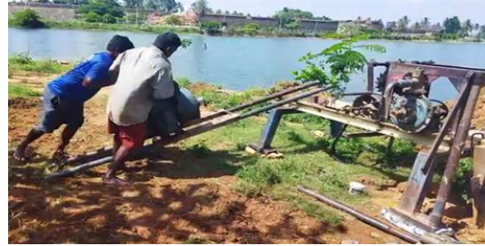
Filter borewell diggers
