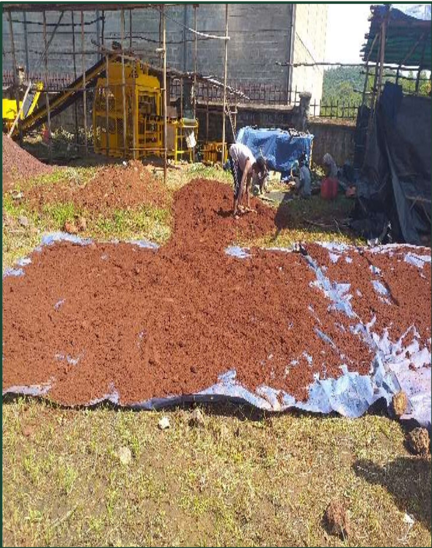
Raw sludge-clay-red ash blend, drying before mixing
