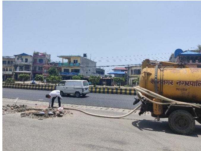
Figure 29: Desludging from manhole by municipal desludging vehicle.
