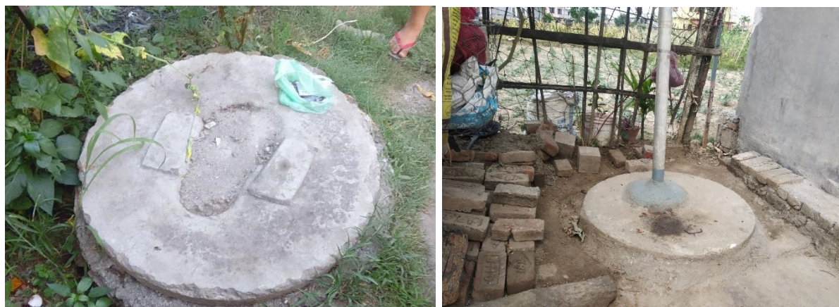
Figure 7: Single pits found in Ratnanagar Municipality
