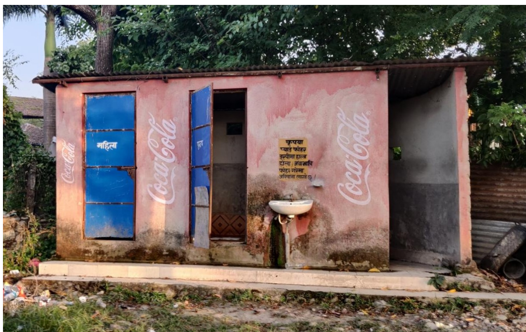
Figure 14: Public toilet B located at Sauraha Bazaar .
