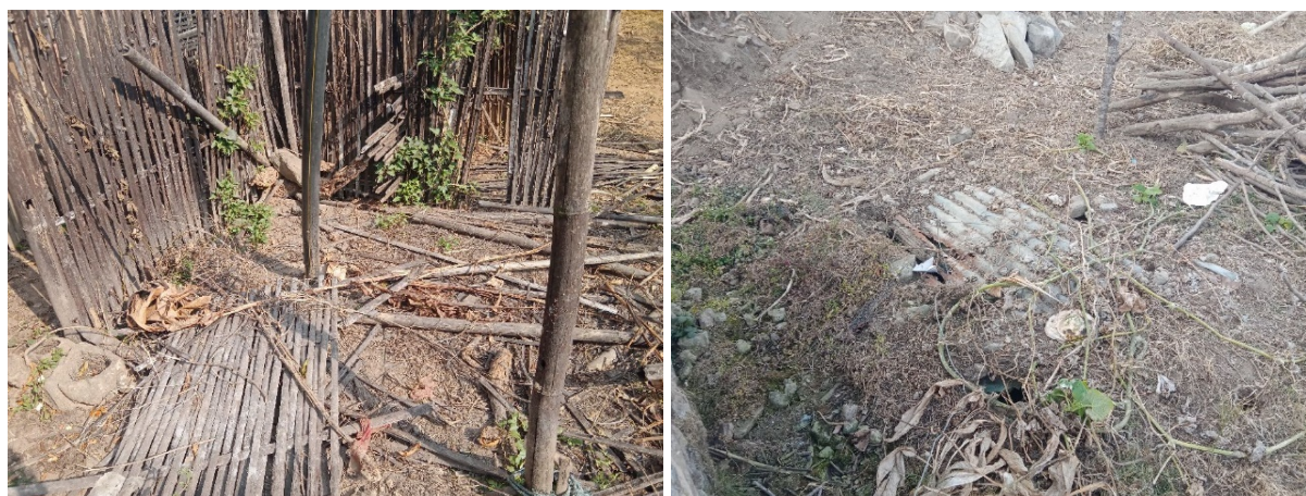
Figure 6: Unlined pits found at households in Bhojpur Municipality.
