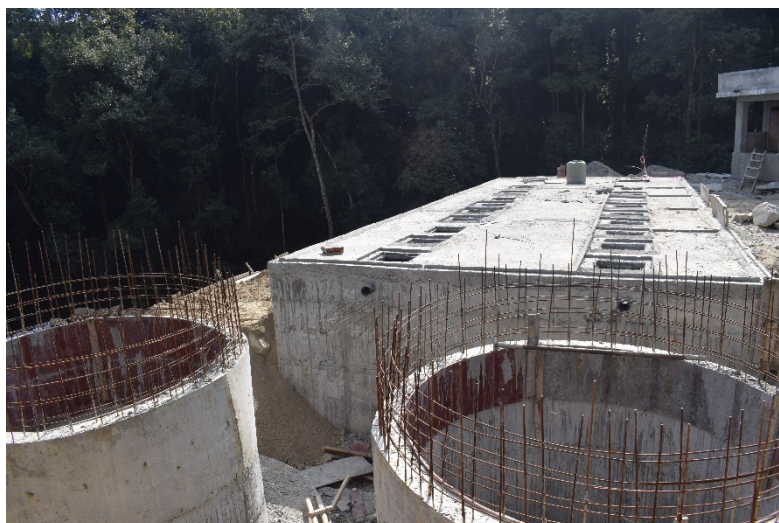
Figure 22: Wastewater treatment plant in construction phase at Bhojpur Municipality.
