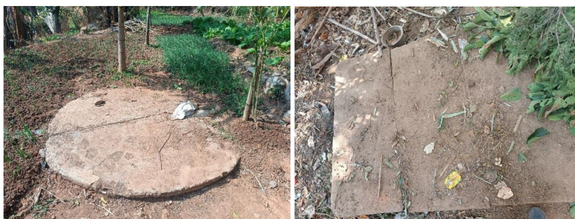
Figure 5: Biogas digesters found at households in Bhojpur Municipality.
