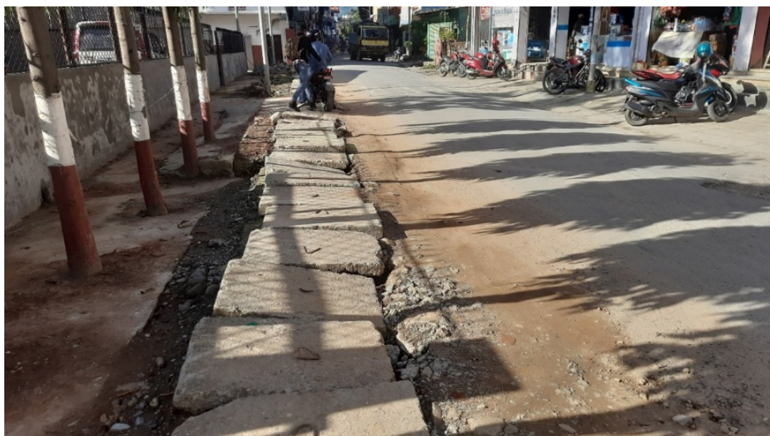
Figure 5: The stormwater drain in Baglung Municipality.
