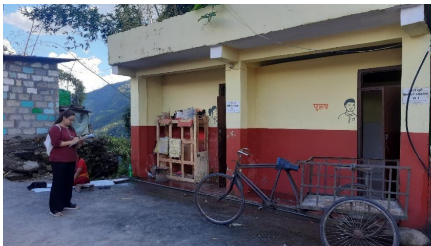
Figure 20: Observation of public toilet at Baglung Municipality.
