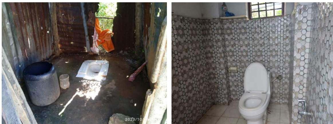
Figure 3: Sanitation technologies at households of Gorkha Municipality.
