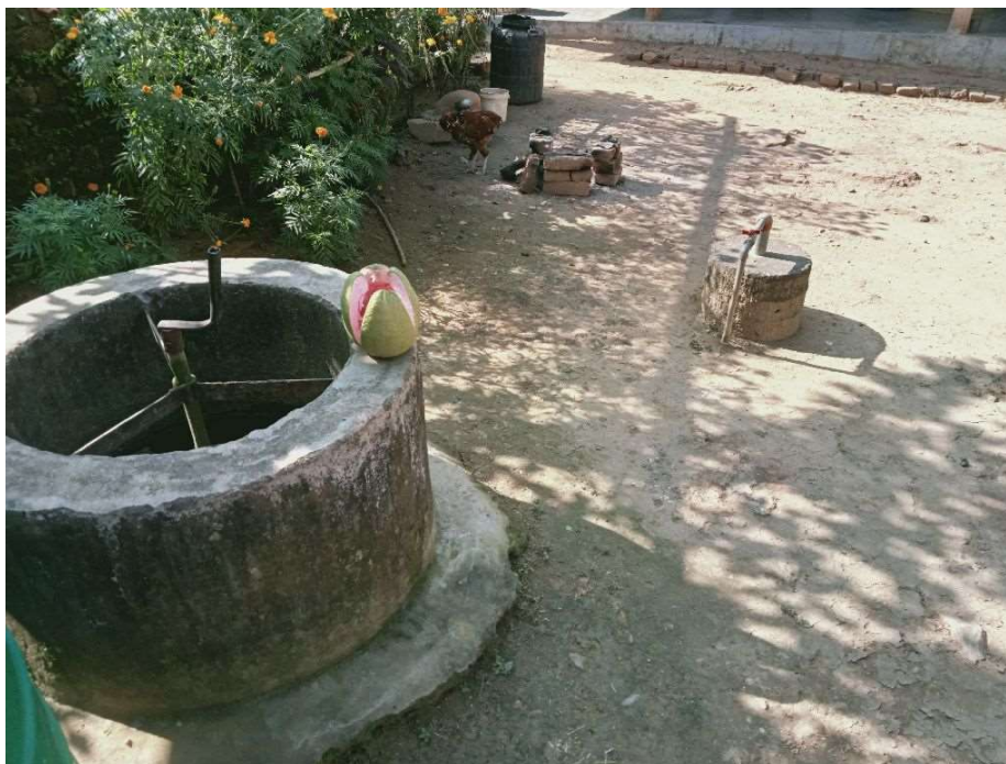
Figure 5: Biogas digester at household of Gorkha Municipality.
