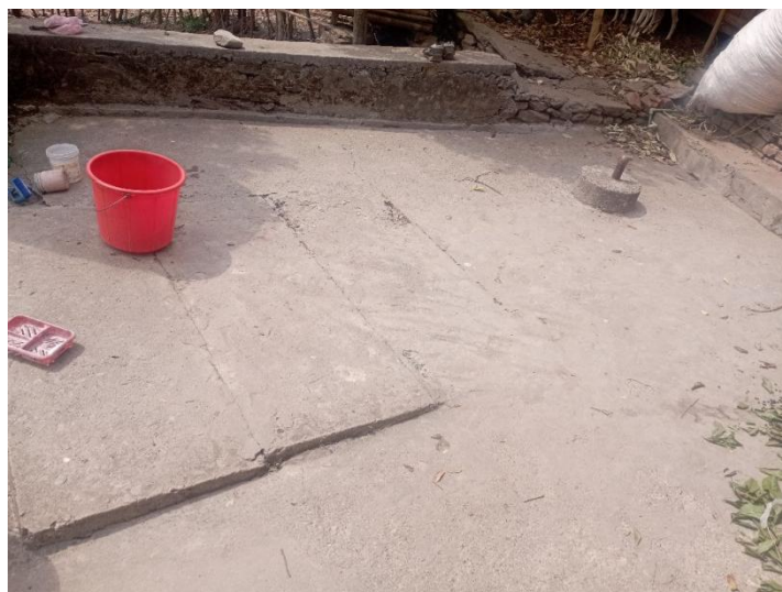
Figure 6: Biogas digester at household of Resunga Municipality.
