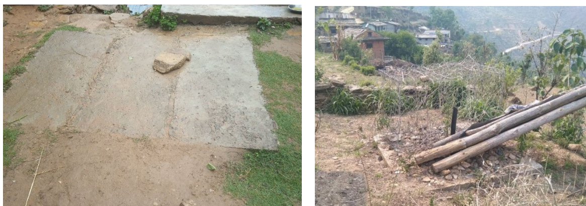
Figure 3: Toilets connected to fully lined tank in households.
