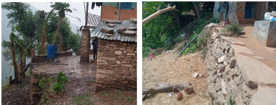
Figure 2: Toilets connected to unlined pits in Bheri Municipality.
