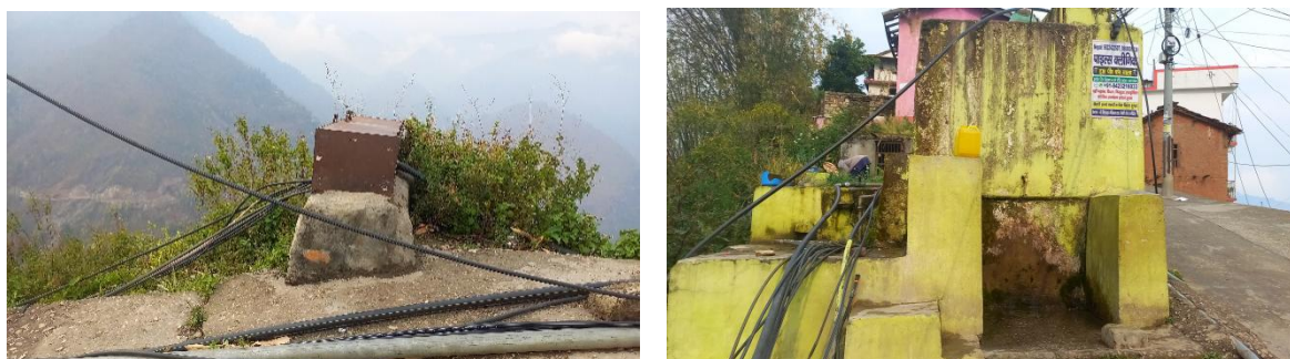
Figure 10: Open pipeline existing within municipality.
