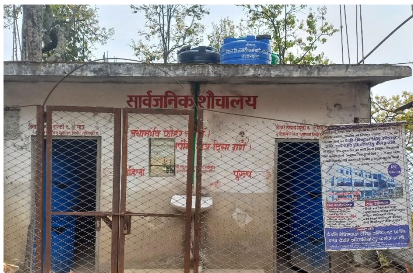
Figure 7: Public toilet in Buspark of Bheri Municipality.
