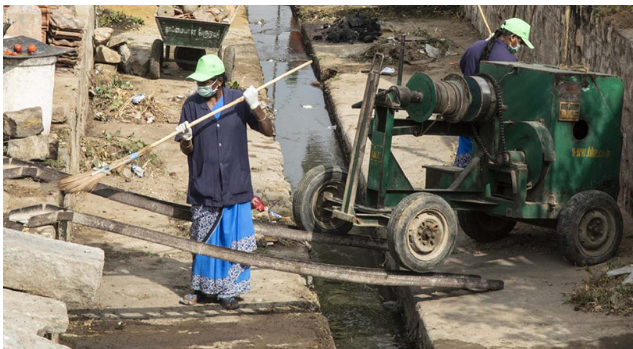
Figure 57. Sanitation workers working in challenging situations
