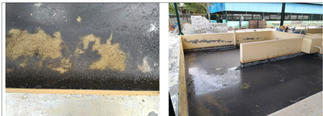
Figure 41. Effect of industrial waste disposed at treatment plant
