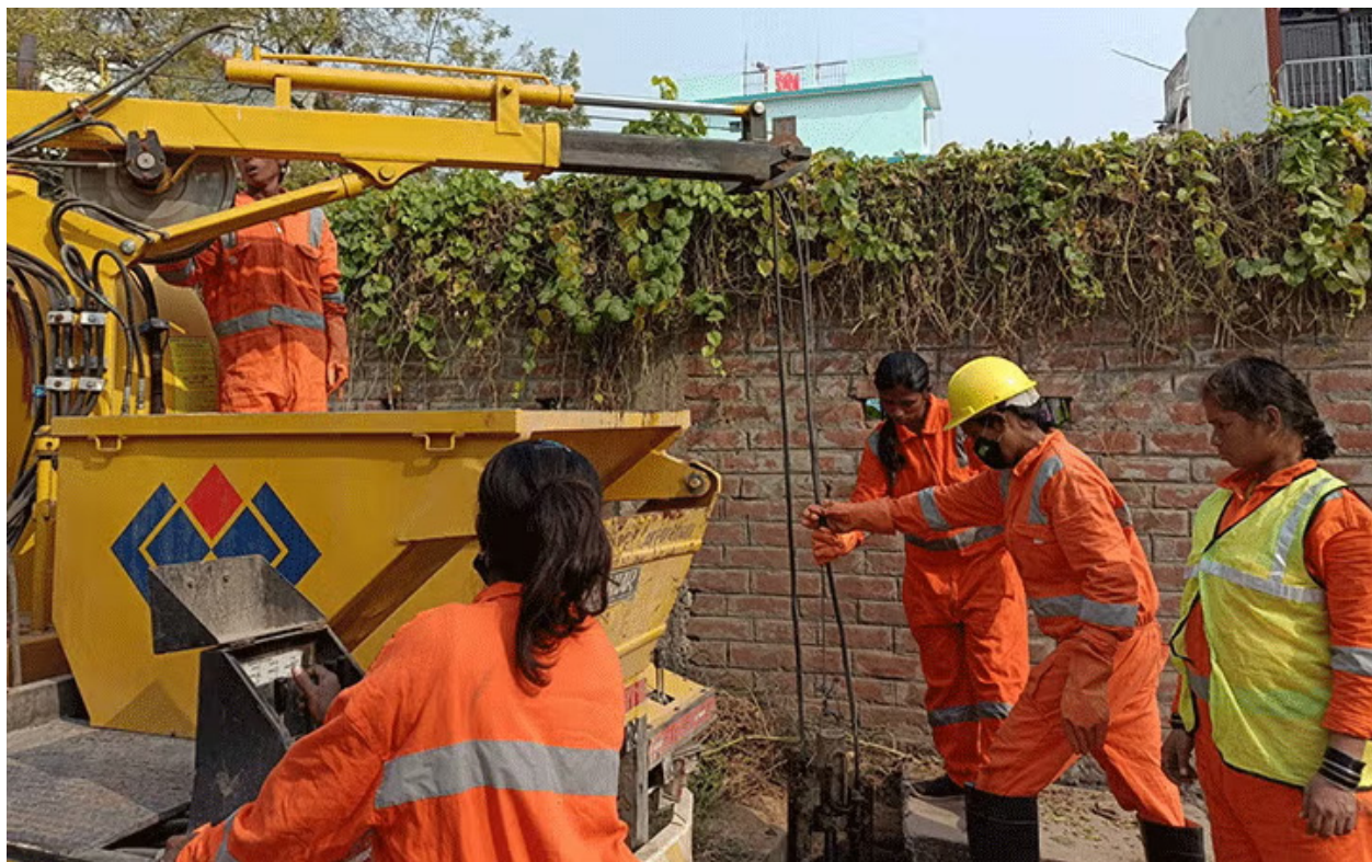
Figure 56. Women sanitation workers in Patna safely clean a sewer using the new mechanized system
