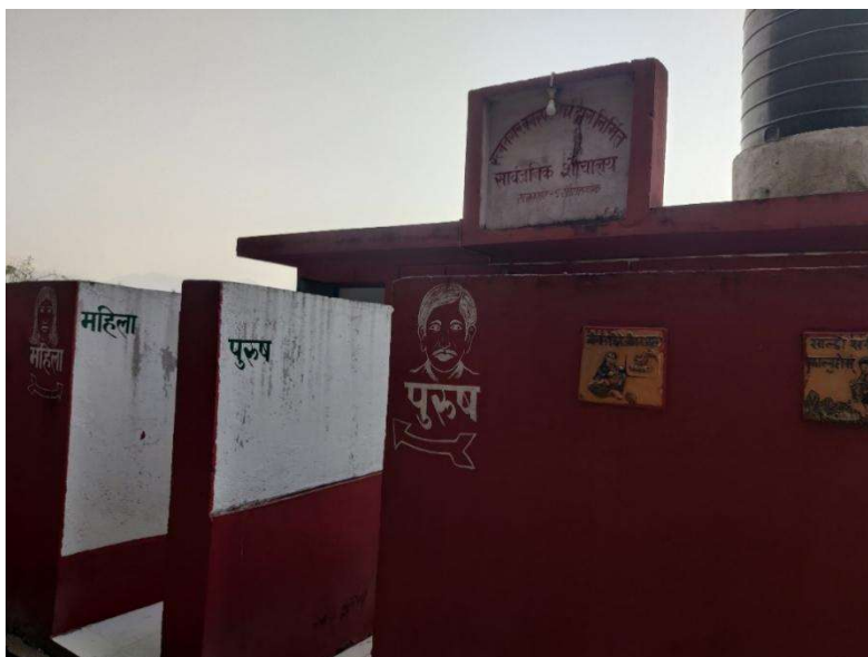
Figure 12: Public toilet located at Saurahachowk .
