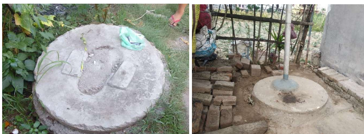
Figure 7: Single pits found in Ratnanagar Municipality
