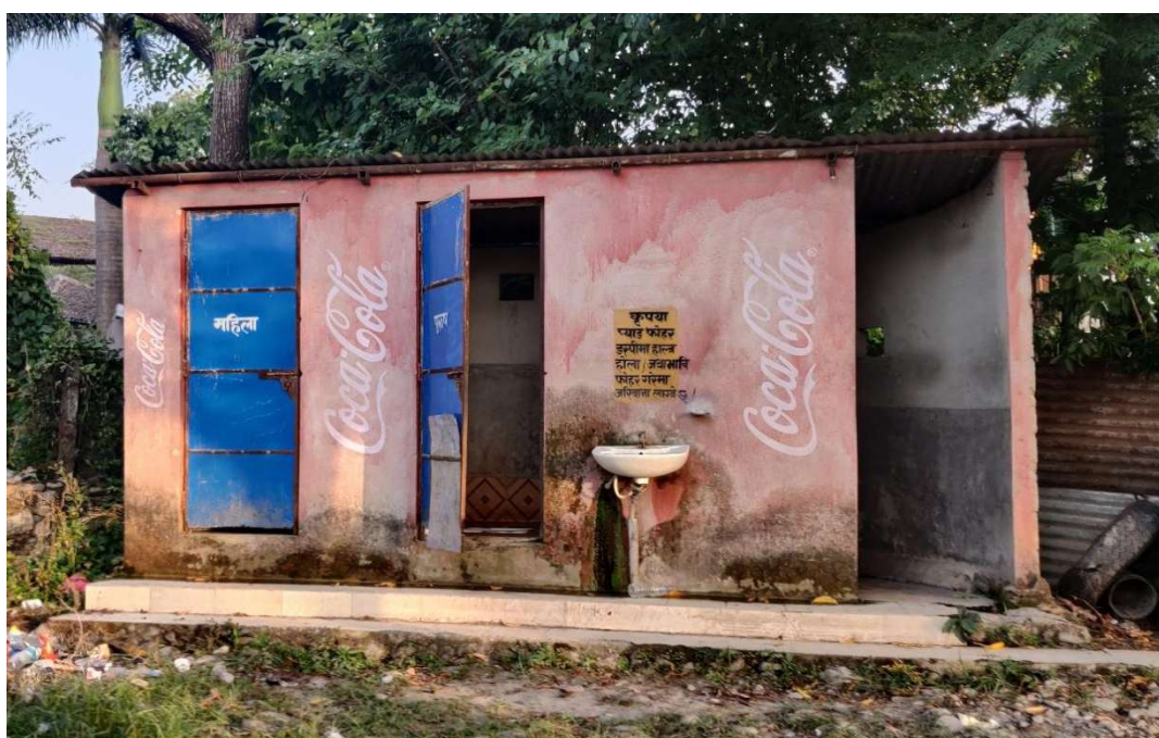
Figure 14: Public toilet B located at Sauraha Bazaar .
