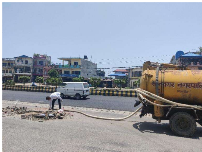
Figure 29: Desludging from manhole by municipal desludging vehicle.
