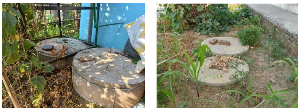
Figure 8: Inappropriate design of twin pits, the distance between two pits is less than 1.2m
