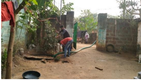
Figure 6: Containments are being emptied by the cesspool operators (Source: Uttama, CFAR. 2025).
