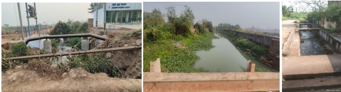
Figure 1: Wastewater discharges through open drains to the Kudiary and Shandapur Canal. (Source: Baijayantimala and Uttama, CFAR. 2025).
