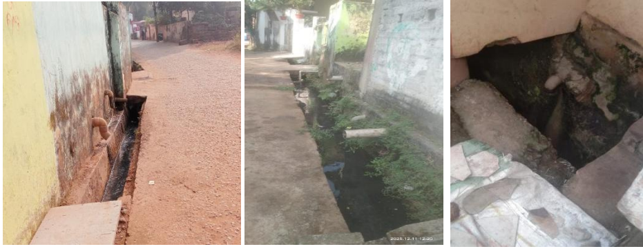
Figure 2: Household toilets are connected to an open drain, Ward Nos. 22 & 13 (Source: Bajjayantimala and Mana, CFAR. 2025).
