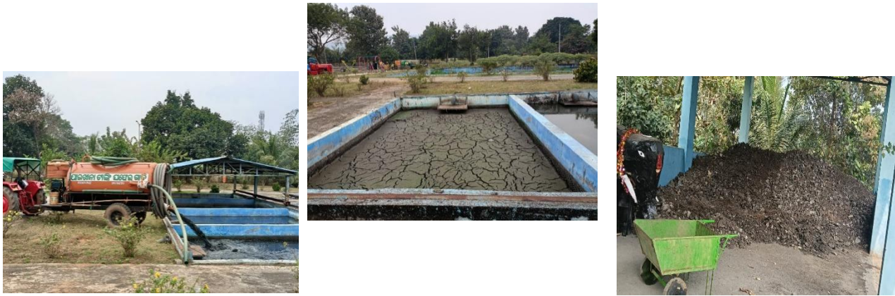
Figure 8: a. Cesspool vehicle unloading septage at the FSTP, b. treated sludge over the drying chamber, c. stockpiled bio-solid (Source: Bulton, Labanya. CFAR. 2025).
