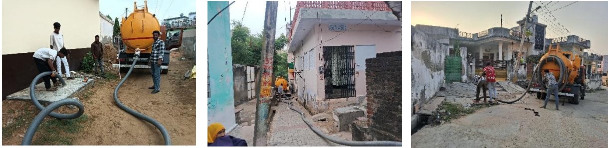
Figure 5: Desludging from the containments with a suction pipe by private cesspool vehicles. (Source: Rajat, Suman & Asha, CFAR. 2025).
