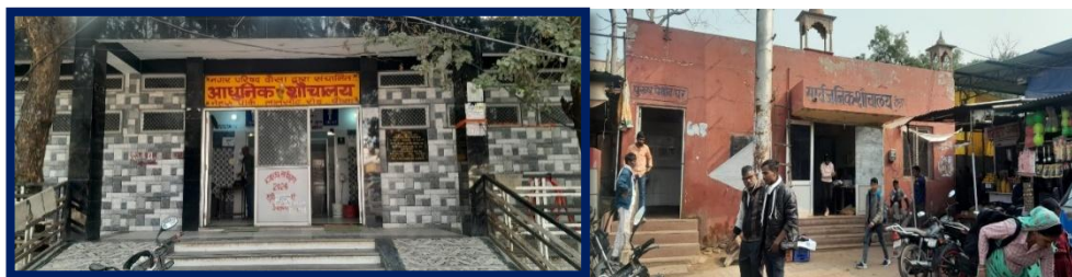
Figure 3: Public/Community toilet facilities in Dausa. (Source: Neelam & Suman, CFAR. 2025).
