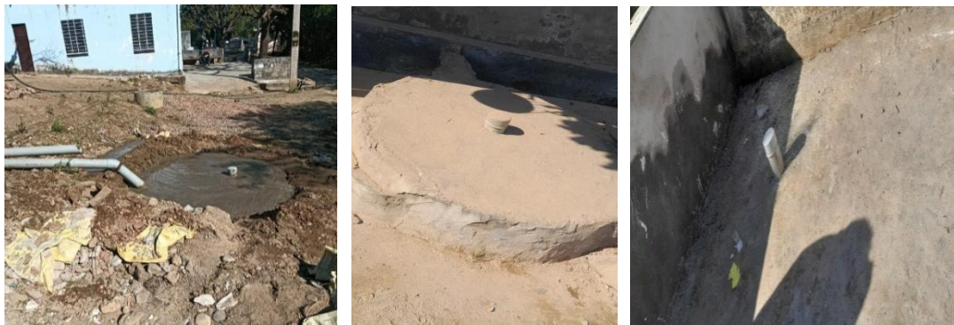
Figure 2: Existing containment structures in Dausa Town. (Source: Rajat & Asha, CFAR. 2025).
