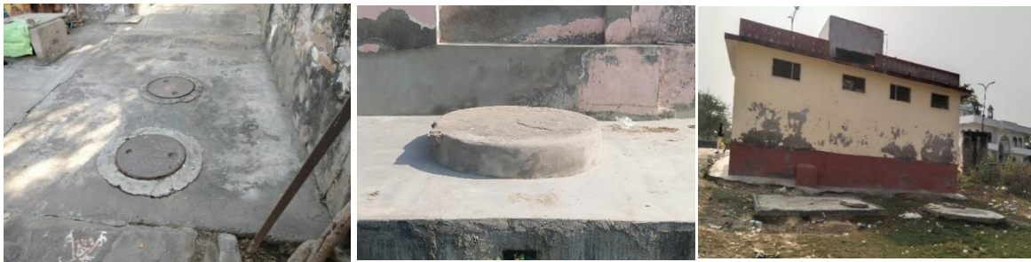
Figure 3: Existing containment structures in Chaksu. (Source: Madhu & Renu, CFAR. 2025).
