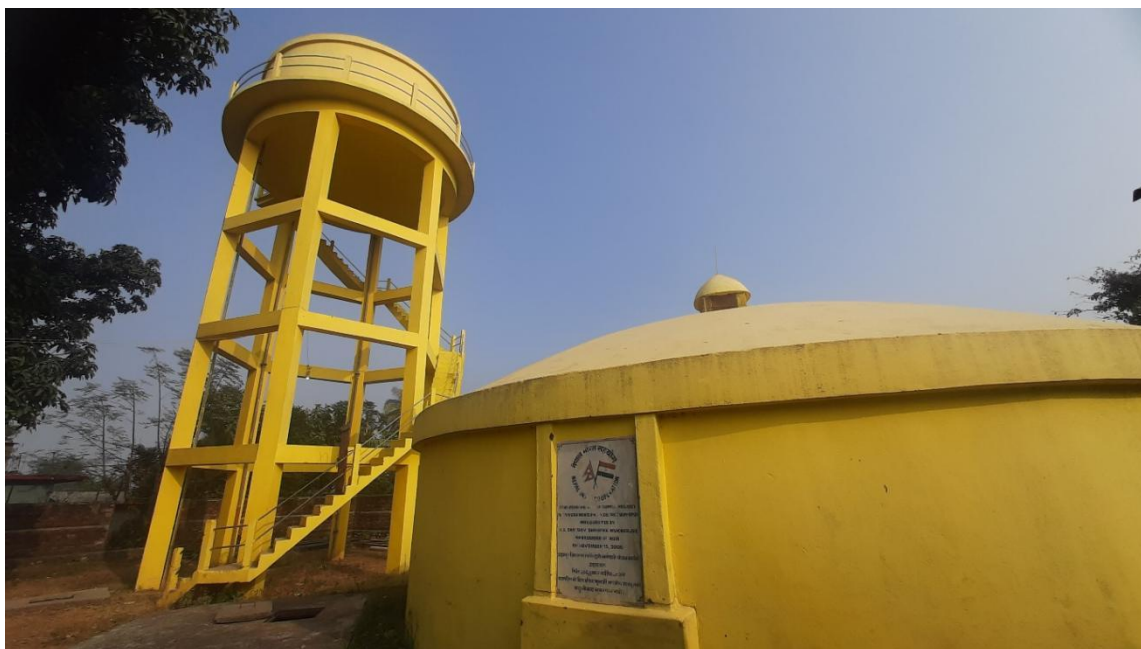
Figure 14: Overhead Tank for Piped Drinking Water Supply System in Triyuga Municipality.
