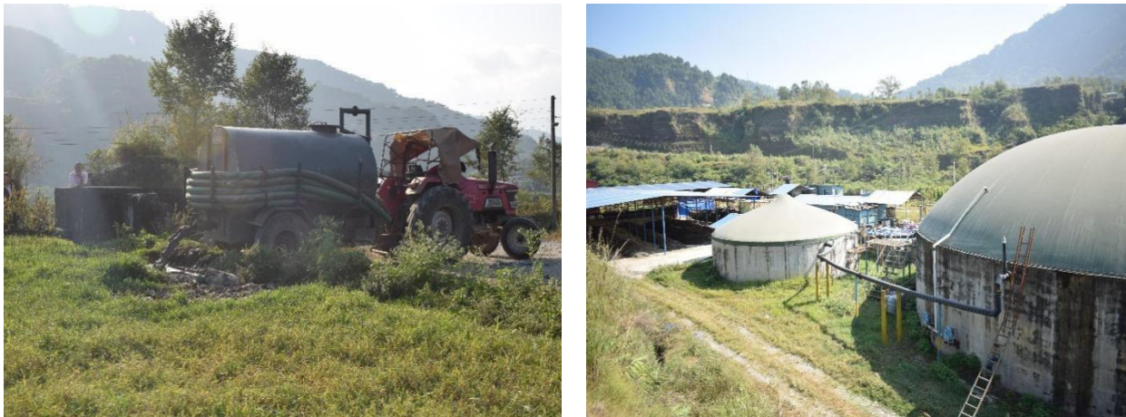
Figure 9: Dismantled Faecal Sludge Treatment Plant (Left) and Gandaki Urja Pvt. Ltd. (Right).
