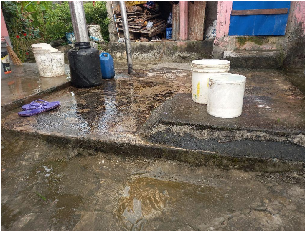
Figure 3: Fully Lined Tank.
