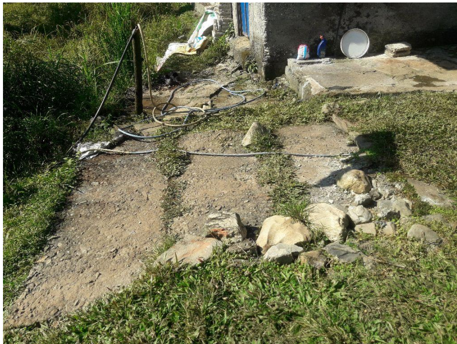
Figure 5: Lined tank with impermeable wall and open bottom installed in the household at Pokhara Metropolitan City.
