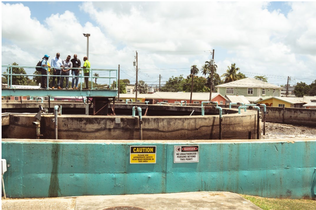
Figure 2 Visit to Bridgetown Wastewater Treatment Plant
