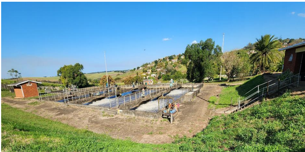
Figure 5: The Ngwelezane WWTW.
