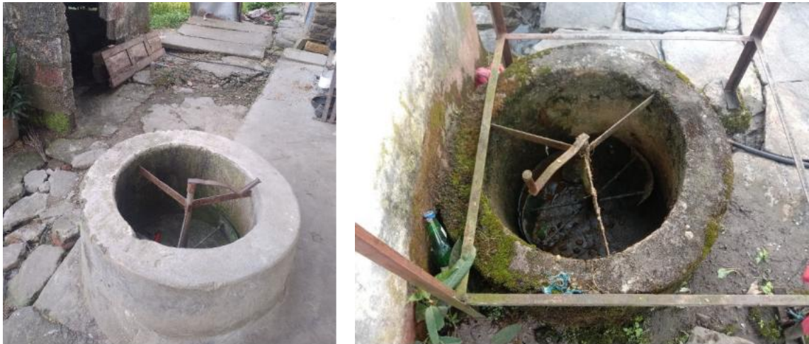
Figure 3: Biogas digester installed in one of the households.
