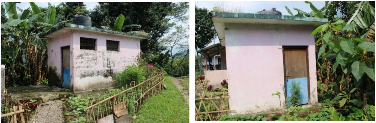
Figure 10: Public toilet located in buspark area.
