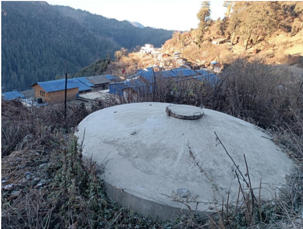
Figure 7: Reservoir tank built by Murma WSUC under USAID project.
