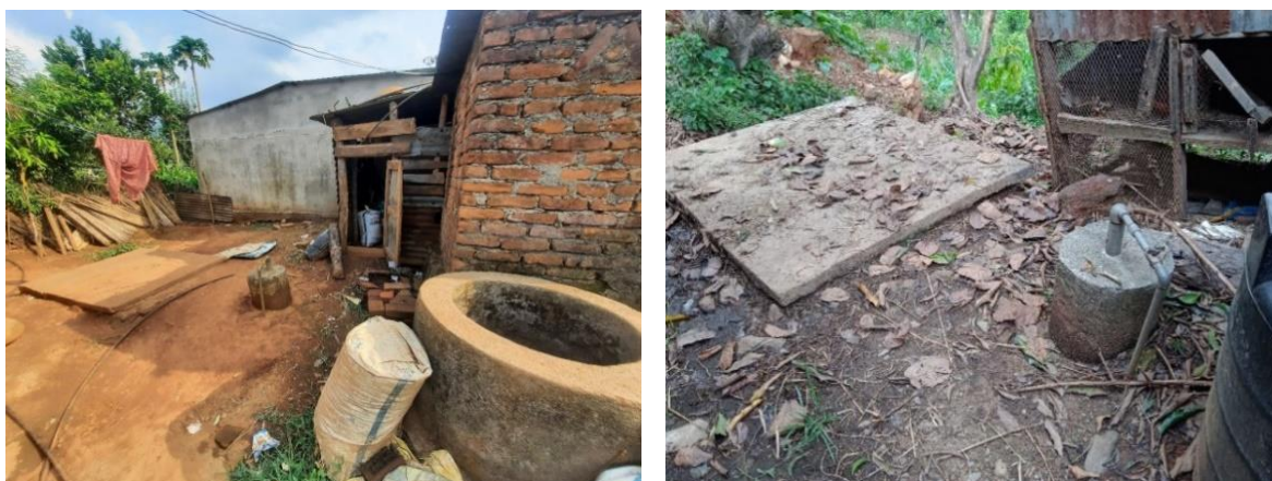
Figure 4: Biogas digester used in Bidur Municipality.
