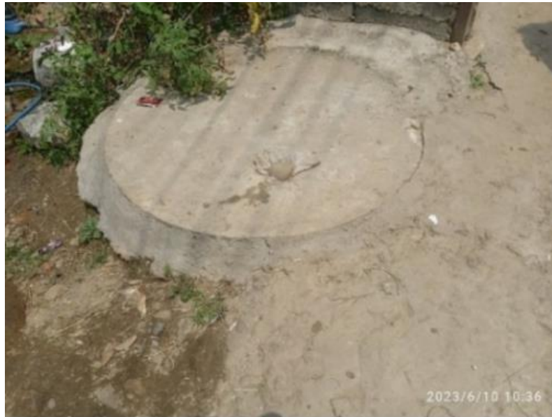
Figure 7: Single offset pit found in Bidur Municipality.
