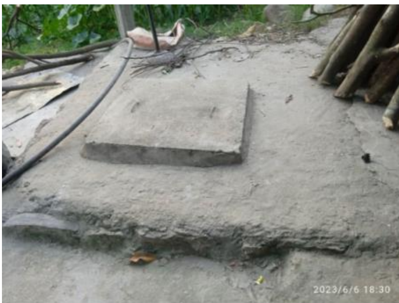
Figure 6: Lined tank with impermeable walls and open bottom at Bidur Municipality.
