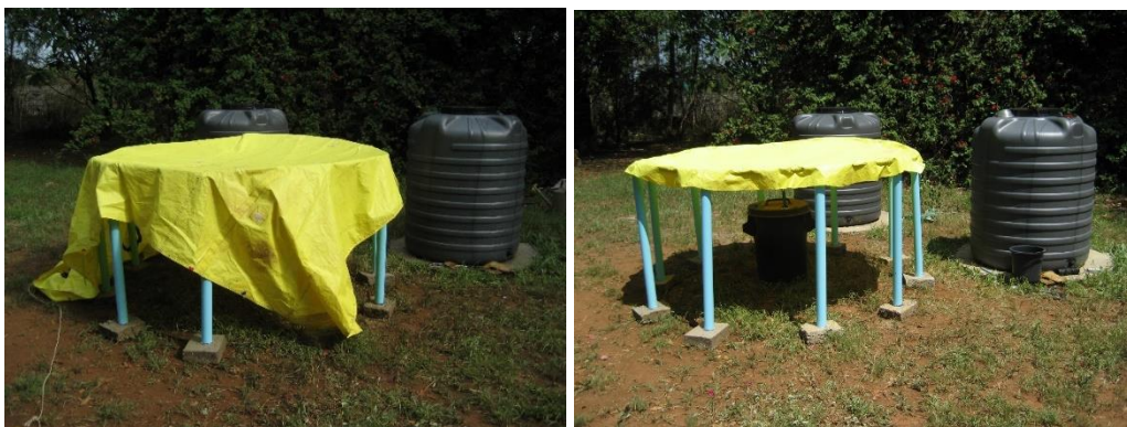
The first of two collectors and the two 1000li tanks which stores the collected water. The material used for the 2 larger “rain catchers” came from a beautiful sail on our cruiser called Aurora. I hesitated to use it at first, but the boat itself being made of wood had been scrapped years ago, but the sail was perfect. It provided enough material to make 2 rain catchers. These were supported by a ring of PVC pipes as shown.
