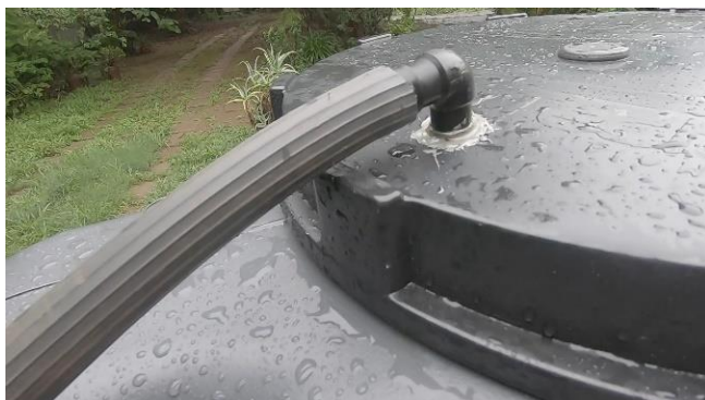
Pipe leading from the lower tank to the upper tank. The pump fitted to the upper tank leads water to various tanks in the garden. The photo on the right shows the pipe leading to one of the 5000li tanks. Water is also pumped to the brick tank next to the 2000li “house tank” which supplies the house with water. There are 3 X 5000li water tanks.
