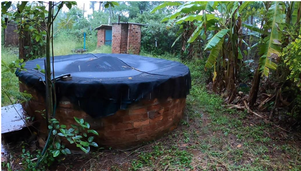
The large brick tank covered with 3 layers of thick shade cloth.
