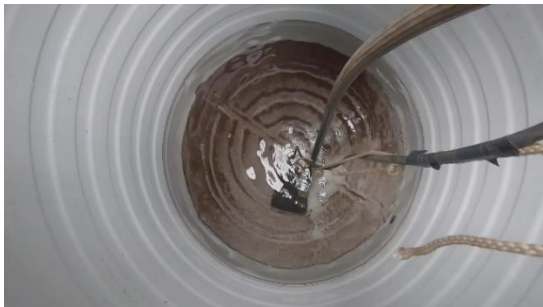
View of lower tank with pump lowered down. And the pipe from the pump leading to the upper tank.
