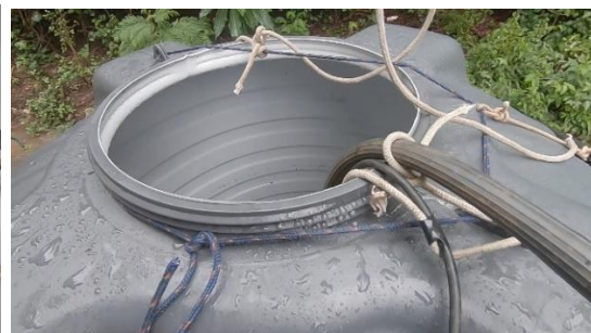
View of lower tank with pump lowered down. And the pipe from the pump leading to the upper tank.
