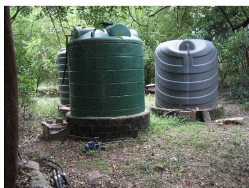
Pipe leading from the lower tank to the upper tank. The pump fitted to the upper tank leads water to various tanks in the garden. The photo on the right shows the pipe leading to one of the 5000li tanks. Water is also pumped to the brick tank next to the 2000li “house tank” which supplies the house with water. There are 3 X 5000li water tanks.
