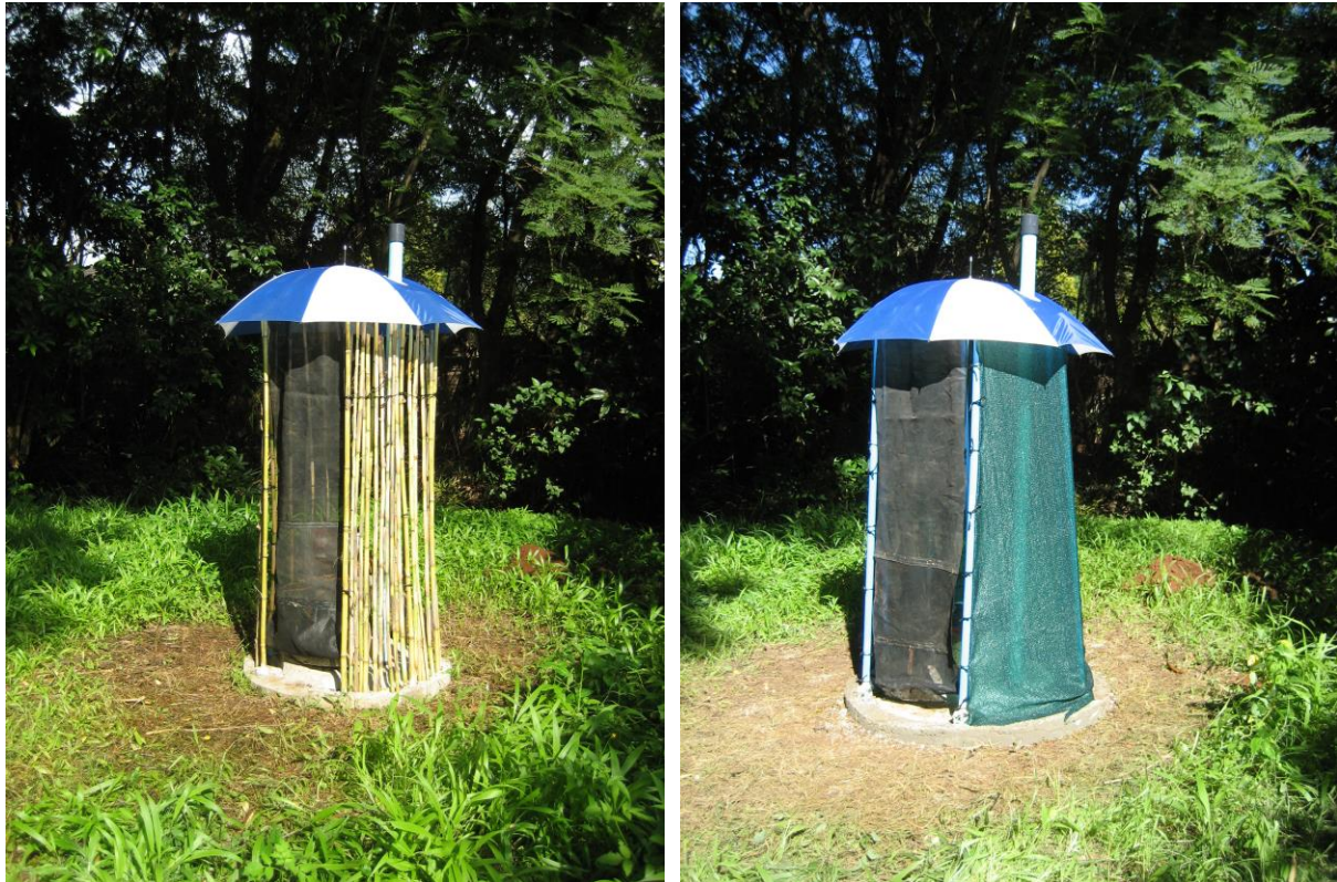
Prototype versions of the ventilated Arborloo designed for children.
