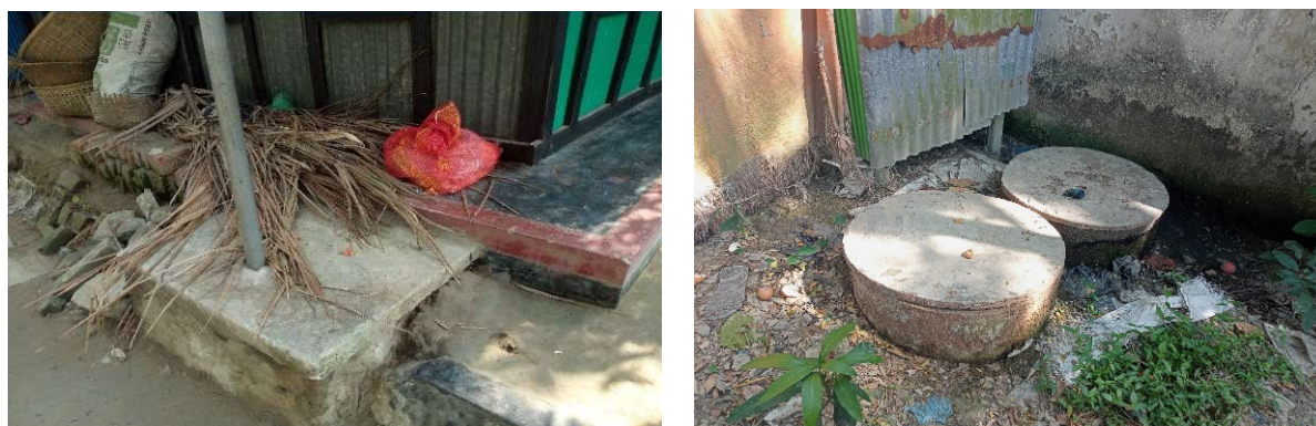
Figure 6: Containment technologies and their connections in Hajiganj Municipality. (Toilet outlets connected to open drains) (Source: Field Survey 2023/ O.CREEDS_ WaterAid Bangladesh).
