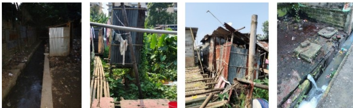
Figure 7: Night Soil Discharged Directly into Open Drains, Water Bodies and Open Drains (Source: Vikash/2024).
