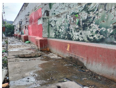
Figure 11: Wall for Nature's Call in a Marketplace (now being dismantled for public amenities) (Source: Vikash/2024-25).
