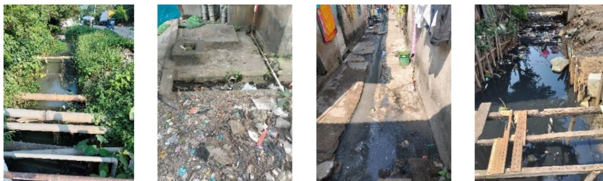
Figure 8: Drains in and around the Slum (Source: Vikash/2024).
