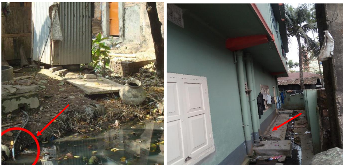
Figure 6: Containment technologies and their connections in Pirojpur . Left: Toilet Pit open to a nearby water body, Right: Toilet pipe connected to open environment. (Source: Feasibility study 2020-21/DPHE).
