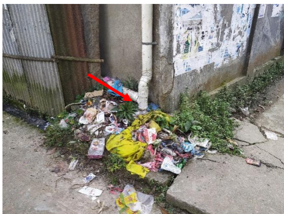
Figure 6: Containment technologies and their connections in Netrokona. Left: Toilet Pit open to a nearby water body, Right: Toilet pipe connected to open environment. (Source: Feasibility study 2020-21/DPHE).
