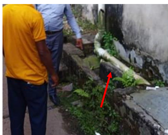
Figure 6: Containment technologies and their connections in Netrokona. Left: Toilet Pit open to a nearby water body, Right: Toilet pipe connected to open environment. (Source: Feasibility study 2020-21/DPHE).
