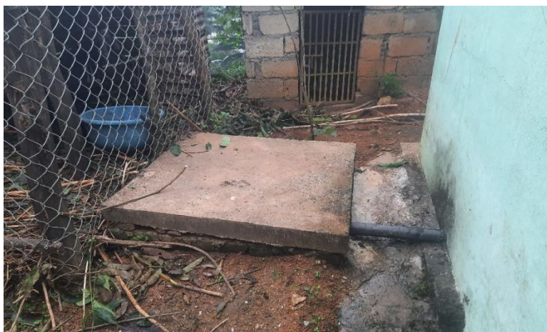
Figure 5: Lined Tank with Impermeable wall and Open Bottom.
