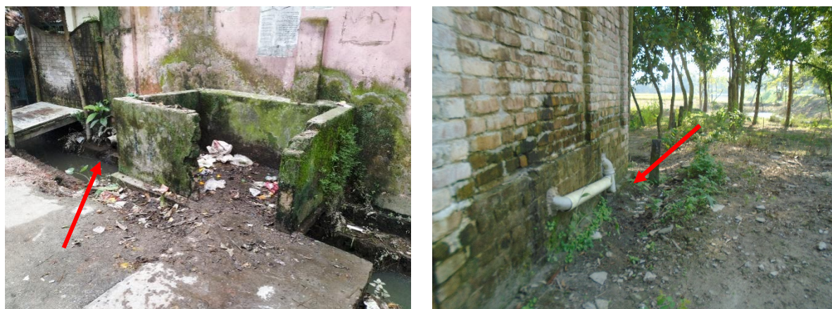
Figure 6 : Containment technologies and their connections in Rangpur. Left: Toilet Pit open to a drain, Right: Toilet pipe connected to open environment. (Source: Feasibility study 2020-21/DPHE).
