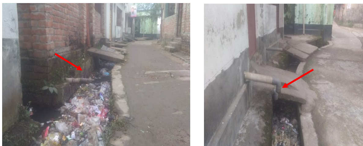
Figure 6: Containment technologies and their connections in Satkhira . Left: Toilet Pit open to a nearby water body, Right: Toilet pipe connected to open environment. (Source: Feasibility study 2020-21/DPHE).
