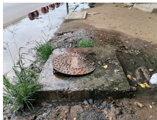
Figure 2: Sewer in poor condition leaking sewage into the street in Yopougon "nouveau quartier" (Source: OUATTARA, 2022).
