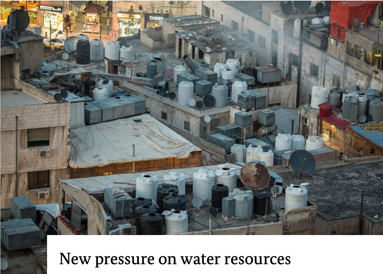
← Water storage tanks on Jordanian rooftops
