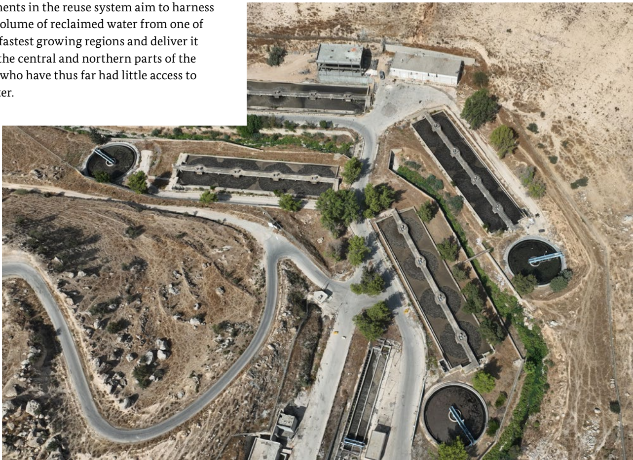
↓ Wadi Al Arab wastewater treatment plant
