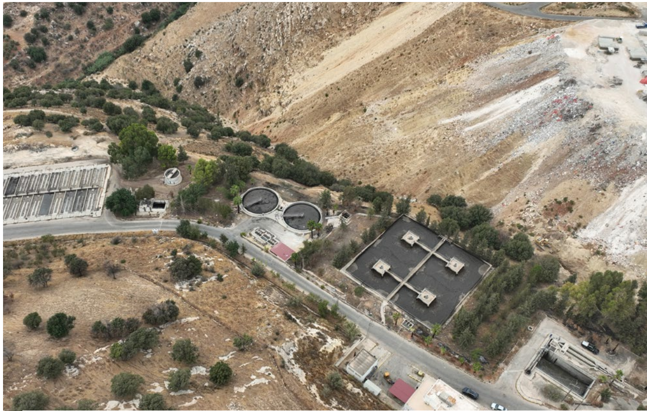
← Fuheis wastewater treatment plant
