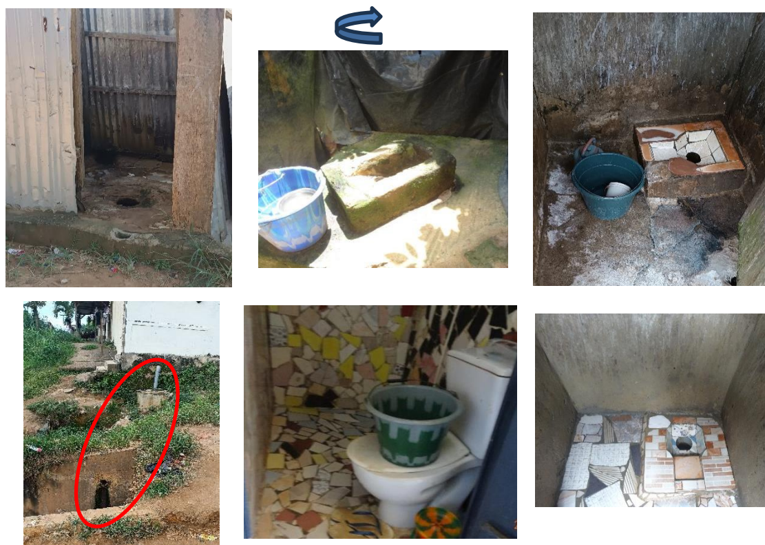
Figure 4: On-site sanitation technologies used by households in Yopougon: A, B) traditional latrines; C, D) Turkish toilets; E) flush toilets; F) anarchic pit connection (Source: TRA, UFHB/CSRS, 2022).
