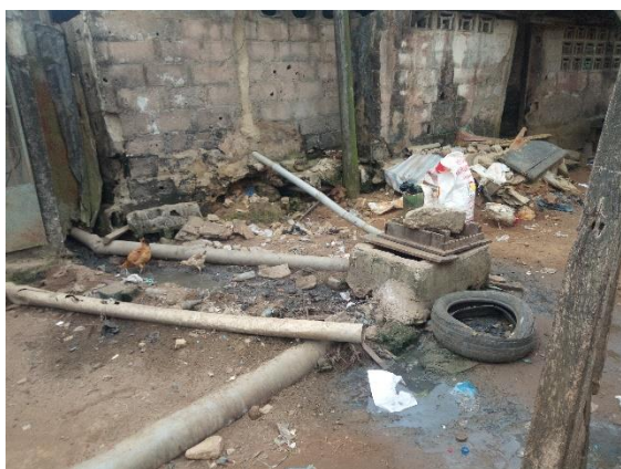
Figure 3: A non-compliant pit leaking fecal matter into the environment in Yopougon "Andokoi" (Source: TRA, 2022).
