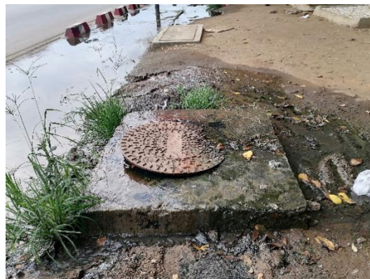
Figure 2: Sewer in poor condition leaking sewage into the street in Yopougon "nouveau quartier" (Source: OUATTARA, 2022).
