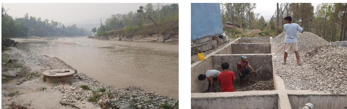
Figure 13: Deep boring sump well nearby Bheri River and filtration unit under construction at Ramghat.
