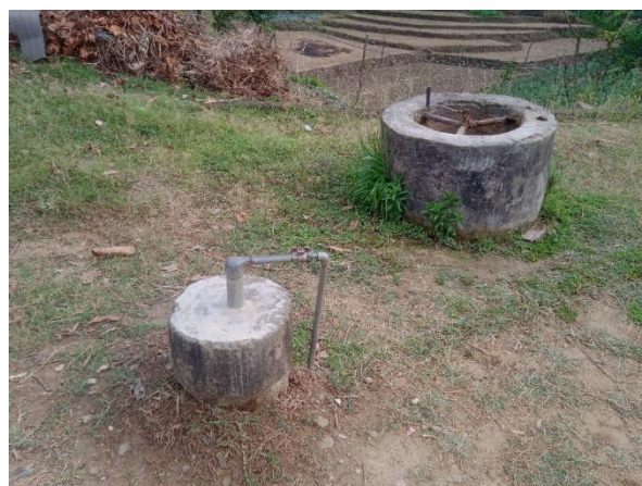
Figure 3: Toilets connected to biogas digester in households.
