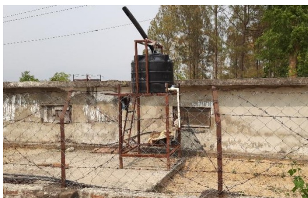
Figure 12: Reservoir tank with automatic chlorination unit.
