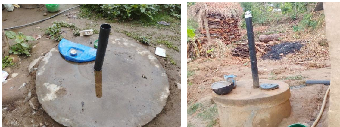
Figure 4: Toilets connected to single pit in households.
