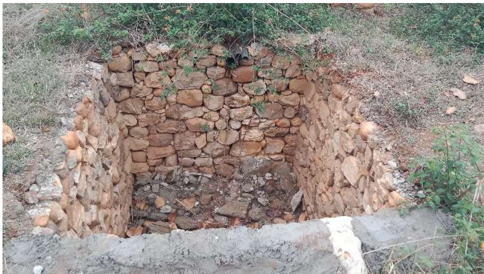
Figure 2: Unlined pit under construction in Bheriganga Municipality.
