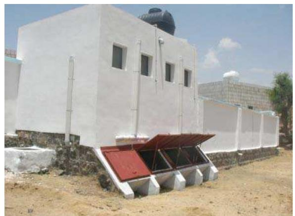
Fig. 3: Urine diversion dehydration toilets at school in Almaraha, showing the red access hatches to the four faeces vaults of the four cubicles (source: GOPA, May 2008).
