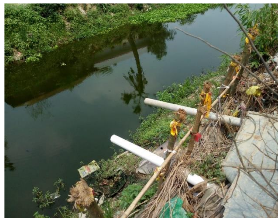
Figure 6: Containment technologies and their connections in Debidwar Municipality (Source: Field Survey 2023/ O.CREEDS_ WaterAid Bangladesh).
