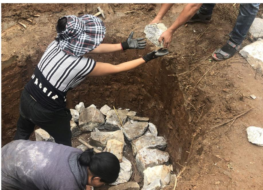
Female masons laying stones for pit toilet construction in Guma Gewog, Bhutan
