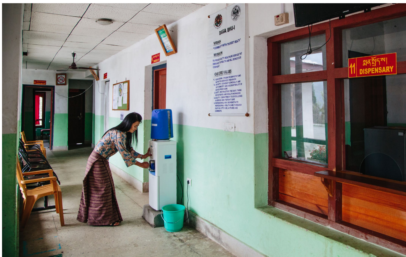
Drinking water for staff and patients at a point of care in a HCF in Dagana district, Bhutan, where SNV has collaborated with the Ministry of Health and other key stakeholders to improve WASH in HCFs as part of their Water for Women project Credit: SNV / Aidan Dockery
