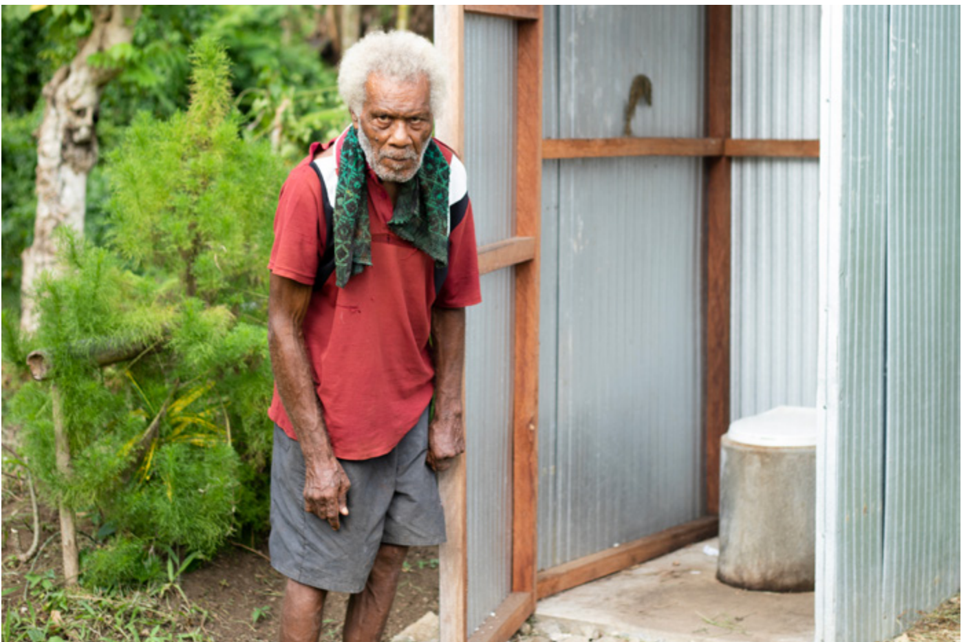
An elderly man stands in front of his new inclusive and accessible latrine, built close to his home with support from Plan International and LLEE through WfW Credit: Plan International and LLEE PNG
