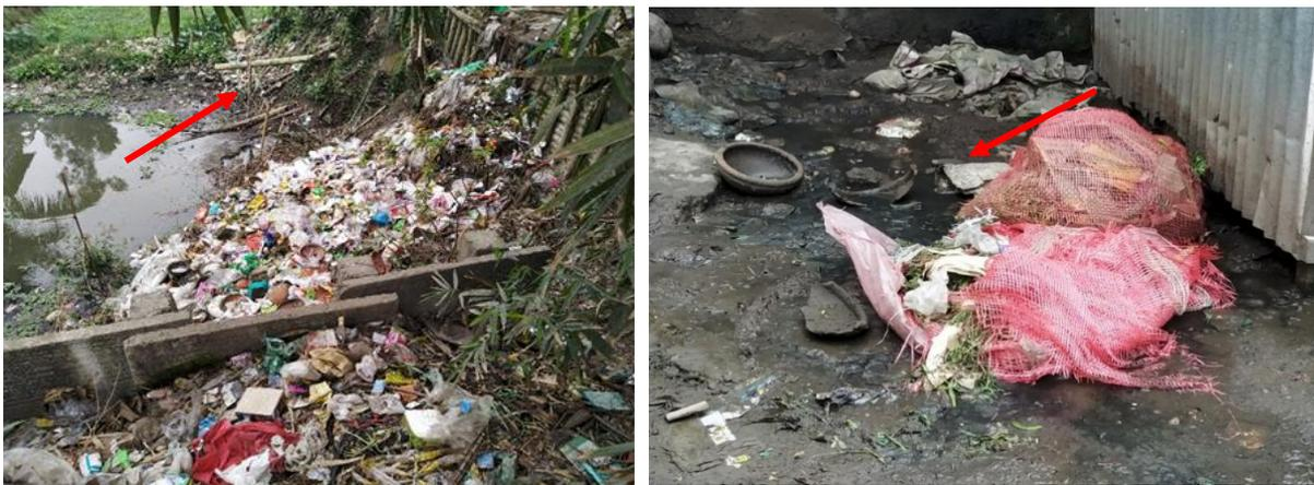
**Figure 6: Containment technologies and their connections in Munshiganj. Left: Toilet Pit open to a nearby water body, Right: Toilet pipe connected to open environment. (Source: Feasibility study 2020-21/DPHE).**
