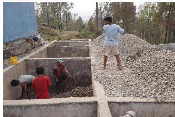
**Figure 13: Deep boring sump well nearby Bheri River and filtration unit under construction at Ramghat.**
