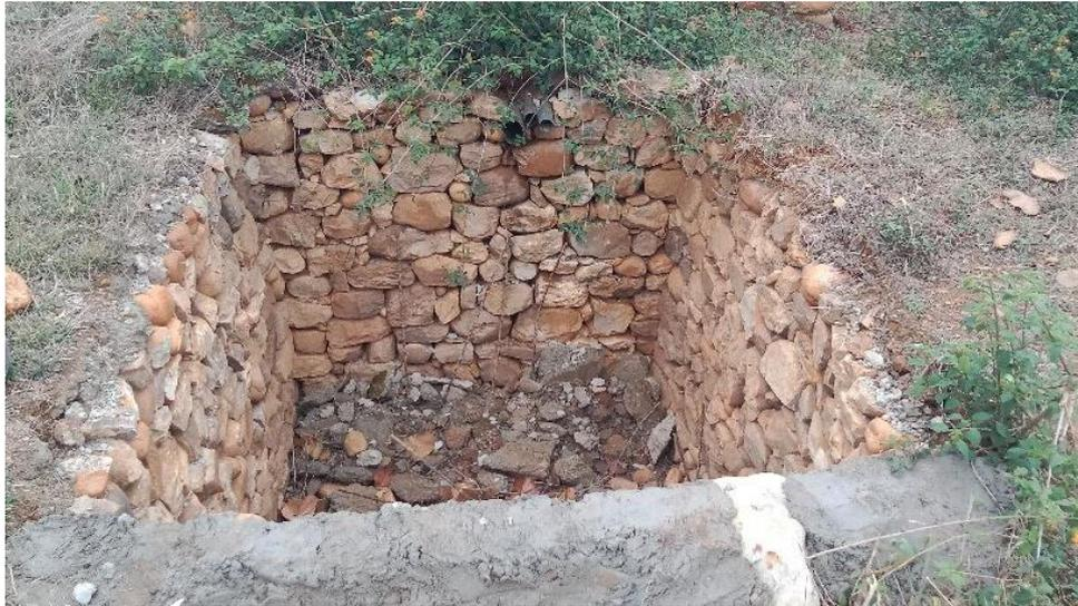
**Figure 2: Unlined pit under construction in Bheriganga Municipality.**
