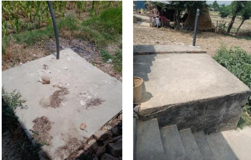
**Figure 3: Fully lined tank built near the farmland in household level.**
