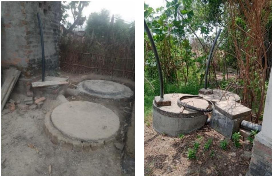
**Figure 5: Twin pits with proper distance as seen in household.**
