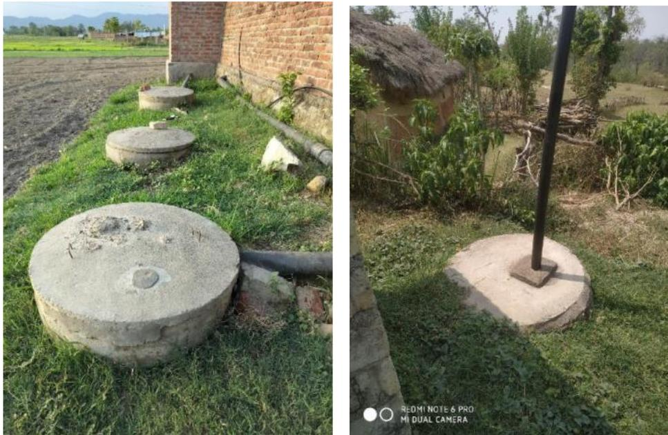
**Figure 6: Two different picture of single containment built in different household.**
