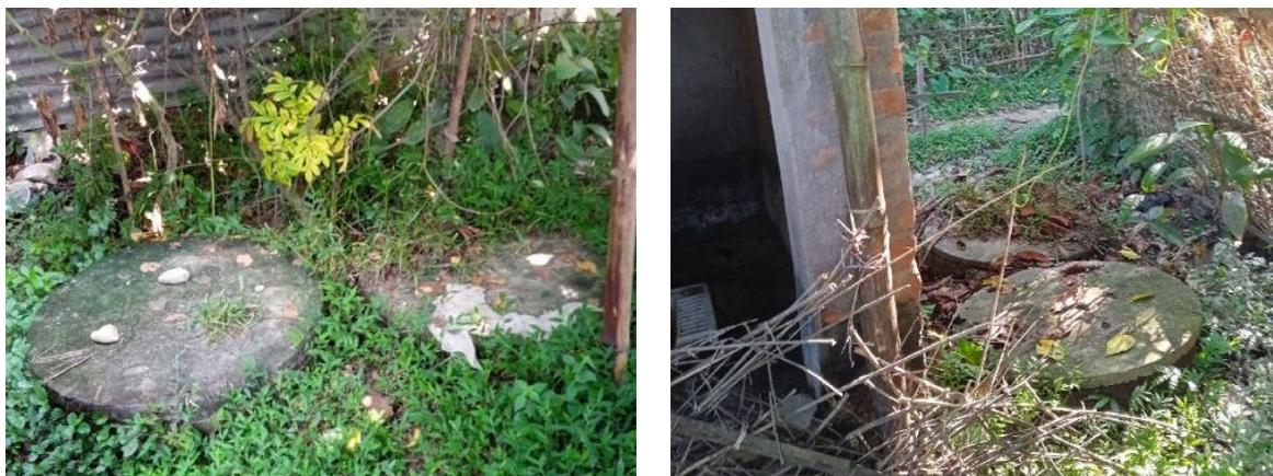
Figure 5: Inappropriate design of twin pits, the distance between two pits is less than 1.2m.
