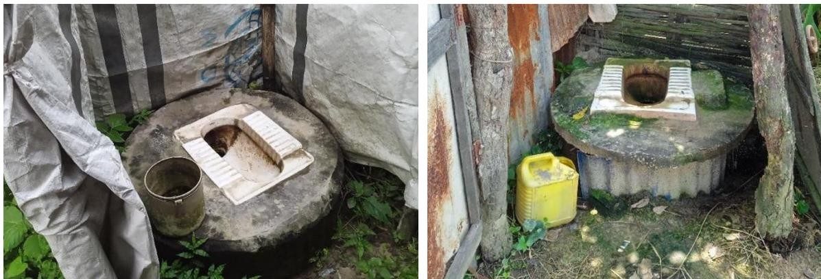
**Figure 6: Types of unlined pits in the municipality.**
